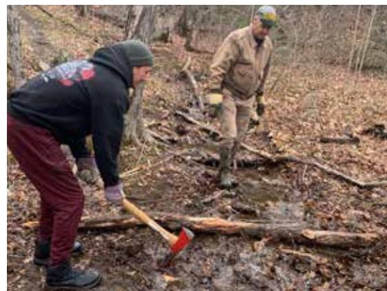
Installing waterbars to deflect water off the trail.
