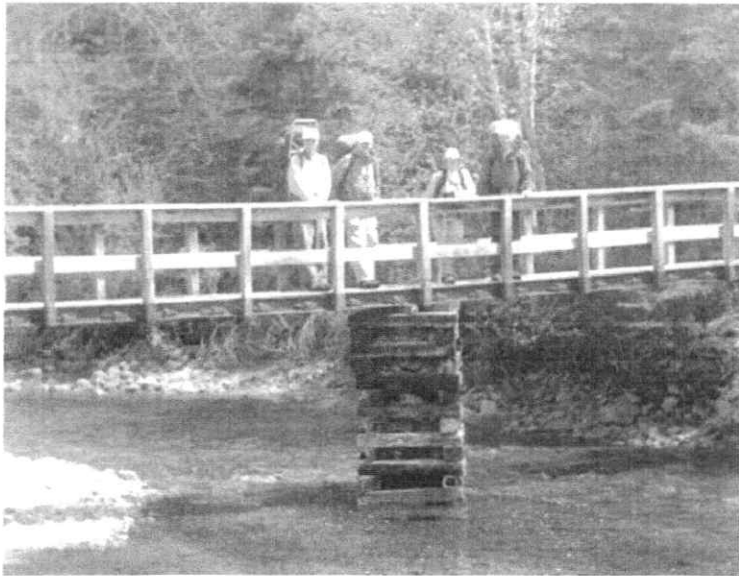
Baldhead River bridge
